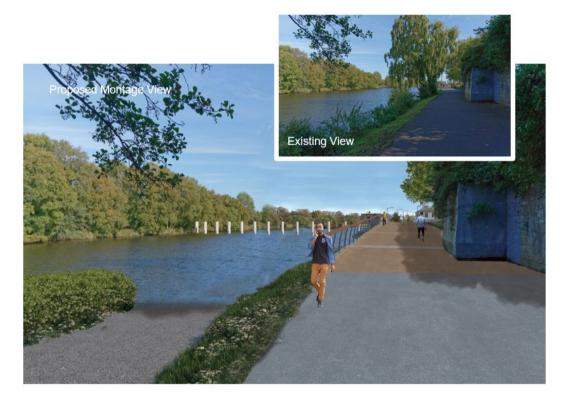
Figure 4.2 Photomontage Showing Proposed Debris Trap
